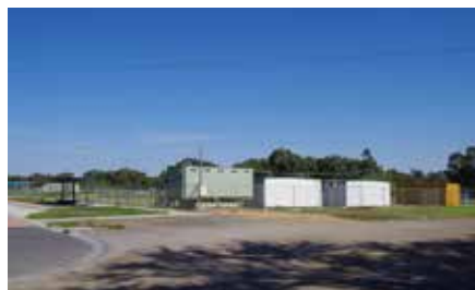
Builders' huts and fencing in place
