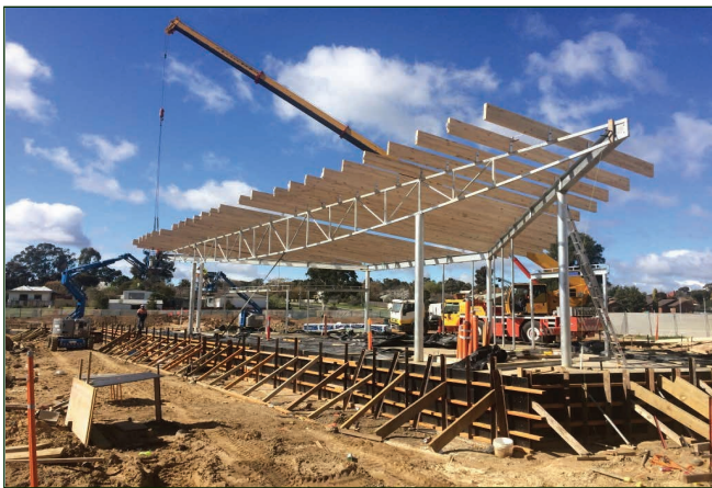
Outreach Shelter under construction
