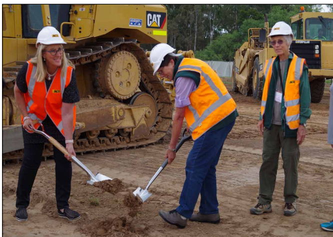
Turning the first sod for the 'Garden for the Future' June 2017
