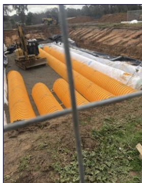
Underground storm water storage
